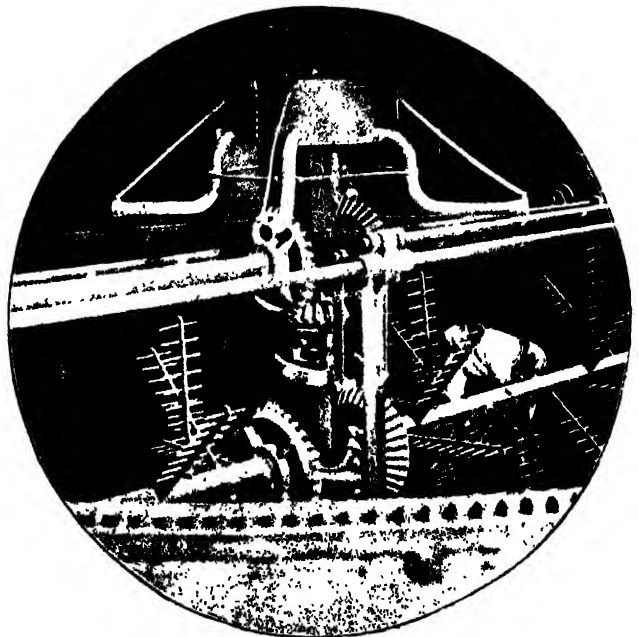
INTERIOR OF MASH TUN (MESSRS. WATNEY'S BREWERY). THE MECHANISM IS SHOWN STATIONARY. THE MAN IS REMOVING ONE OF THE SLOTTED PLATES THROUGH WHICH LIQUID DRAINS FROM GRAINS.
